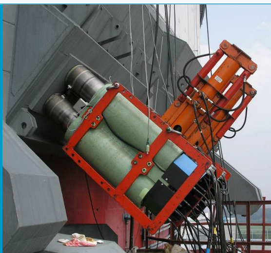
Pre-stressing of tendons and prestressing force checks (9,5 or 9,1 MN)
